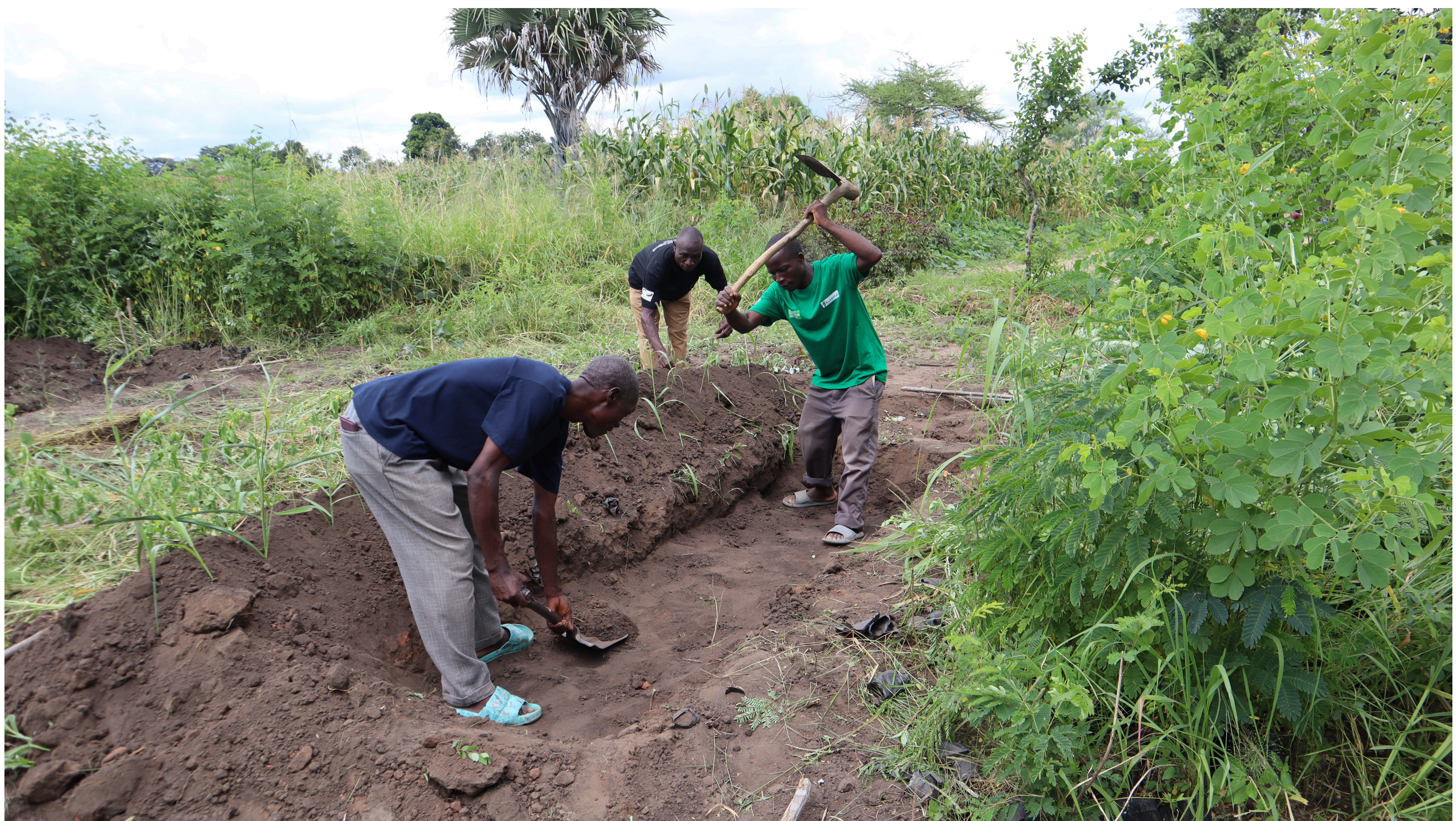
Construction of a swale in progress
